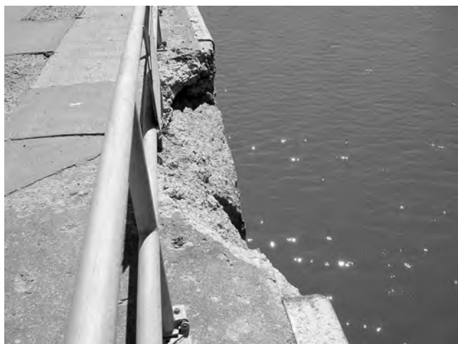
Picture showing the LaGrange Lock crumbling side wall
